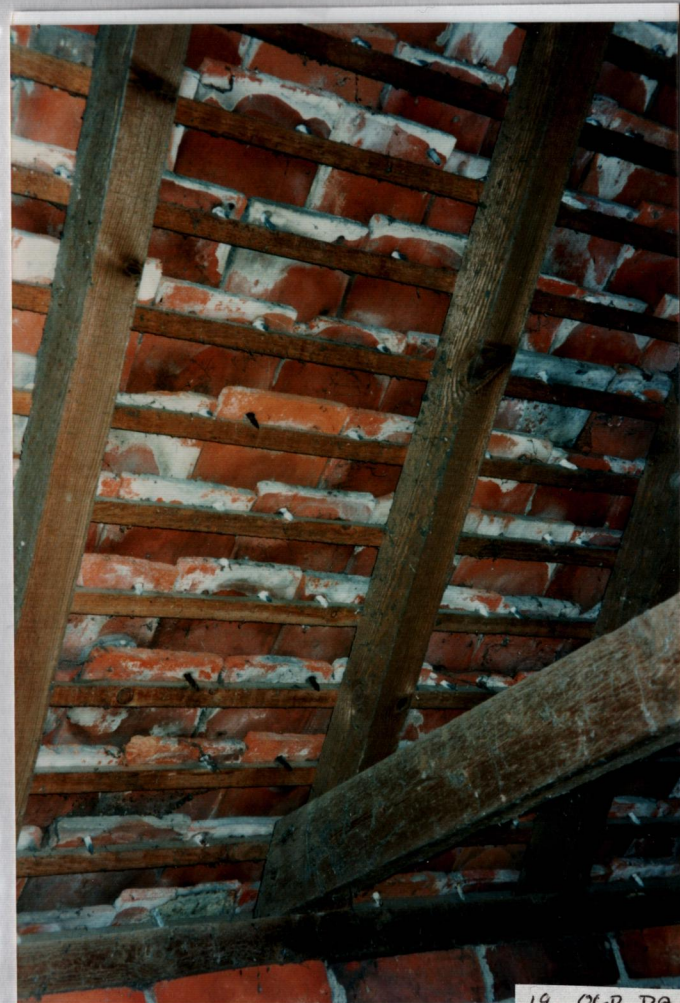
19. OLD DAIRY RAFTERS
