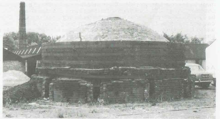
A circular down-draft or beehive kiln with ten stoke-holes and underground flues to a separate chimney. Warfield, 1965
