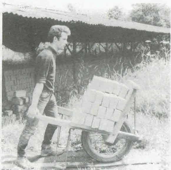
Taking the dried bricks to the kiln on a crowding barrow
