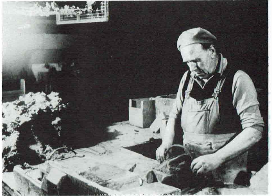
The sequence of hand-moulding. ABOVE: Cutting off the excess clay with a wire bow. BELOW: The full mould is lifted off the stock board and the brick turned out on to a pallet.
