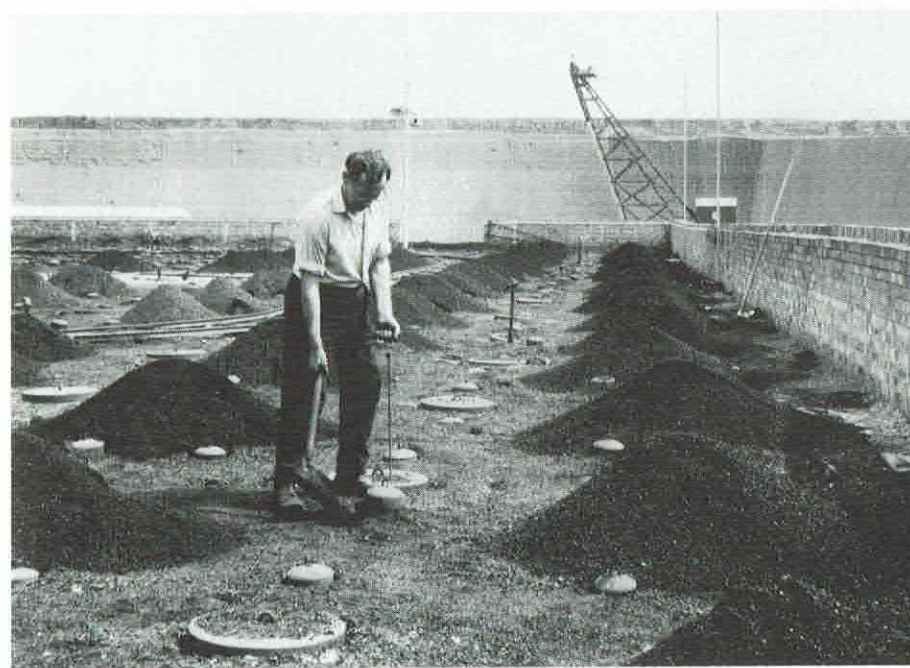
BELOW: Feeding a continuous kiln for Fletton bricks with coal. The small covers are the feedhole caps; the large covers give access to the chamber offtake and inlet bell-dampers in the hot air flues.
