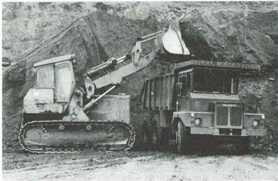
BELOW: Loading weathered clay into a dumper truck from a stockpile.
